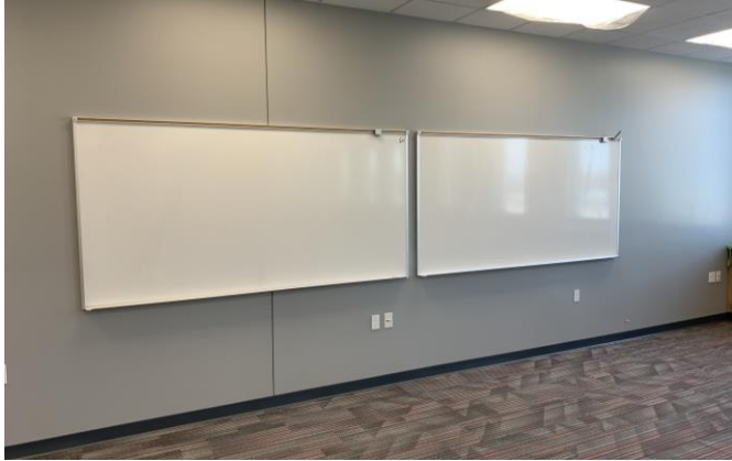
White boards going up in classrooms 01/23/2023
