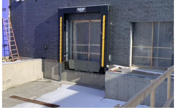
Completed loading dock 01/23/2023
