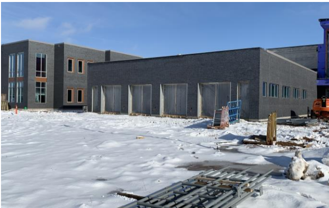
Completed brick on the auto shop 01/23/2023
