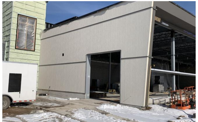
Exterior siding on the weight room 01/23/2023
