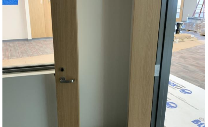
Wood doors are hung in North classroom wings 01/23/2023
