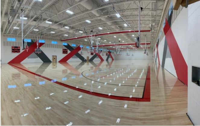
Auxiliary gym completed wood floor 01/16/2023
